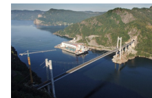
E39 Lyngdal - Flekkefjord Improved connection Kr,Sand - STV Highway 38,500 m - 1.2 BNOK 2011-2012
